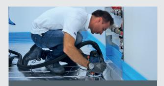
After marking the track you wish to create with a felt-tip pen, proceed to make it with a cutter or, better still, with a common electric DIY milling machine for polystyrene.
