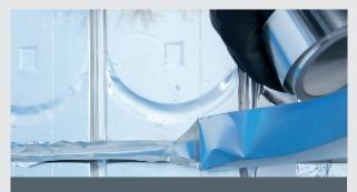
Insert the aluminised adhesive tape supplied by RBM into the track created, in order to restore the aluminised surface layer. Take care to ensure that the tape adheres well to the panel.
