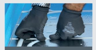
It is imperative that the pipework remains well below the surface of the panel. Apply aluminised adhesive tape on the bends or where necessary to hold the pipe in place.
