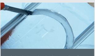
At the bends, the track is already prepared, so all you need to do is cut through the surface layer of aluminium, freeing the underlying housing created for the pipe.
