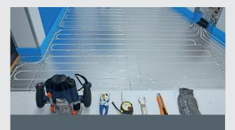
Before laying the flooring, carry out the system leakage test, as required by the standard.
