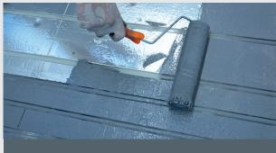
Prior to applying ceramic flooring or cement-based substrates (glued parquet or resilient flooring), apply RBM MF by Mapei epoxy primer and then the bonding primer.
