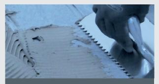
Glue the panel to the substrate with suitable adhesives. For this operation, we recommend MAPECONTACT by MAPEI® reinforced bi-adhesive tape or polyurethane adhesives such as FERMACELL or similar.
