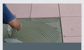
Bond ceramic or natural stone tiles with suitable adhesives such as ELASTORAPID by MAPEI® or similar.
