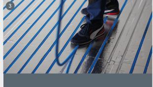
Now you can begin the installation of the radiant circuits, following the properly drawn up installation diagram.
