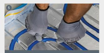
The pipe must absolutely remain well embedded under the surface of the panel. Apply aluminized tape to the bends or where needed to hold the pipe in place.
