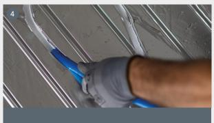
At the bends the track is already prepared, so it will be enough to cut the surface layer of aluminum, freeing the underlying preformed housing for the pipe.
