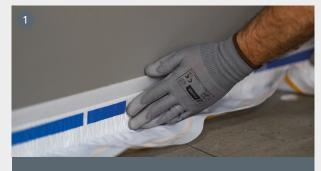
Lay the perimeter edge for the absorption of expansion of the system. This element must be applied on the walls along the entire perimeter of the rooms affected by the system.
