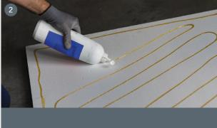
Glue the board to the substrate using KILMA FUTURA AD glue.
