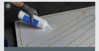
Glue the board to the substrate using KILMA FUTURA AD glue.
