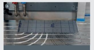
Cutting a new track/guide for the pipe: it may be necessary to make a new track on site to complete one or more circuits or to create new ones.
