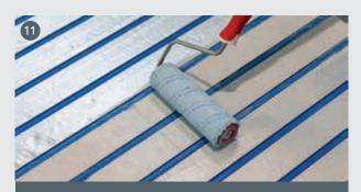
Before applying ceramic tile flooring or cement-based substrates (glued parquet or resilient flooring), apply RBM MF by Mapei epoxy primer and, thereafter, adhesion primer.
