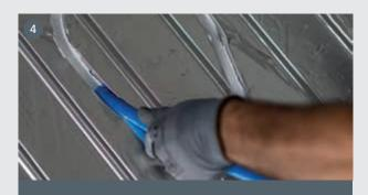
At the bends the track is already prepared, so it will be enough to cut the surface layer of aluminum, freeing the underlying preformed housing for the pipe.
