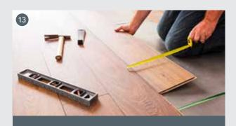
With "floating parquet", no primer will be required but, before laying the parquet with its fabric/nonwoven backing layer, spread a layer of PE.
