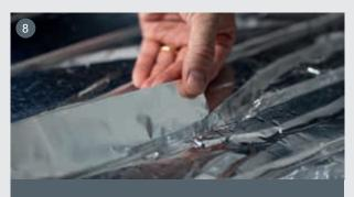
Insert the aluminized adhesive tape provided by RBM into the trace made, in order to restore the aluminized surface layer. Take care to ensure that the tape adheres well to the panel.
