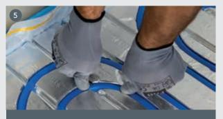
The pipe must absolutely remain well embedded under the surface of the panel. Apply aluminized tape to the bends or where needed to hold the pipe in place.
