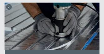
After marking with a marker the track you wish to create, proceed to make it with a cutter or, better yet, with a common DIY electric polystyrene router.
