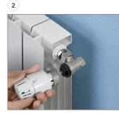
2. Position the polymer spacer onto the valve's body by centring the cap's hexagon (**this operation is necessary only for the 3087 series** thermostatic head - the spacer is supplied as a kit with the thermostatic head).
