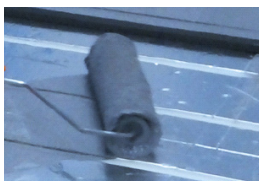
Ceramic covering installation
